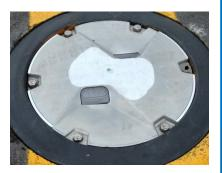
Determine if base is L867B or L868B cut energy to fixture if applicable
